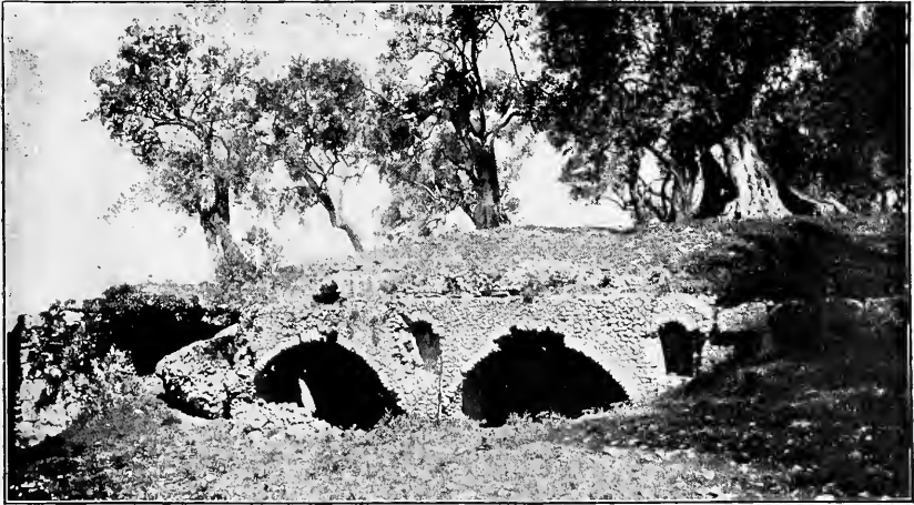
Sand and Pebble Catch-tanks near Tivoli. Dimension-stone aqueducts of Marcia at either end of the tank built of small stone; opus incretum . The arches are chambers of the tanks.
